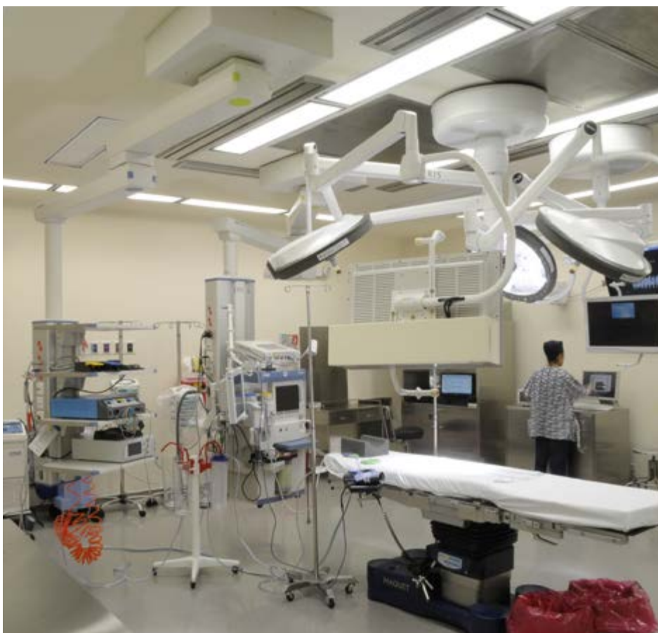
At a new delivery suite at Poole Maternity Hospital, UK, Sikagard®-205W (Sterisheen®) - a high performance surface coating that would meet stringent infection control procedures, was used on the walls and ceilings of the operating theatres.
