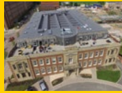
SINGLE PLY ROOFING
