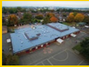
LIQUID APPLIED ROOFING
