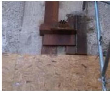
Tie-back (anchoring) of the retaining wall: Not a uniform and continuous substrate, or requires a temporary recess for tie-back.
