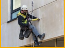
JOINT SEALING
