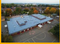
LIQUID APPLIED ROOFING
