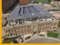
SINGLE PLY ROOFING
