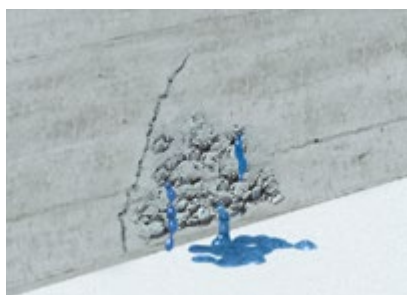
SEALING AND WATERPROOFING OF CRACKS AND VOIDS
