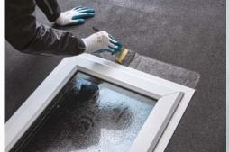
Evercryl is a resin based, fibre re-enforced\* roof repair compound which is effective on all common roofing surfaces, giving instant roof repairs even in the wet and on wet surfaces. May also be applied in frosty conditions down to -5°C.
