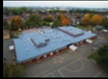
LIQUID APPLIED ROOFING
