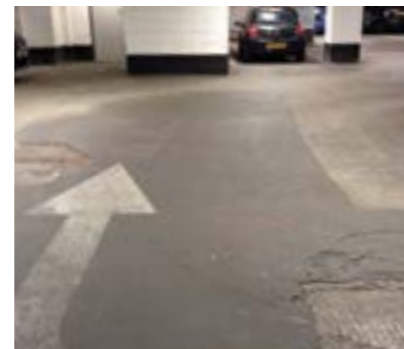
POOR QUALITY REPAIRS
