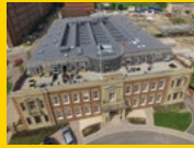
SINGLE PLY ROOFING
