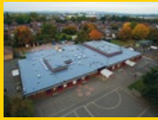
LIQUID APPLIED ROOFING
