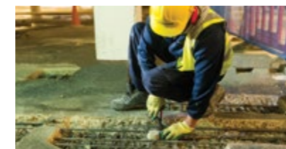
EMBEDDED GALVANIC ANODES
