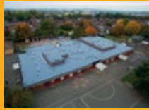
LIQUID APPLIED ROOFING
