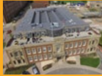
SINGLE PLY ROOFING
