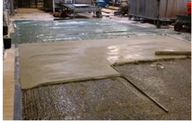
FRIDAY EVENING: Application of the bonding layer and the cementitious fast curing Sikafloor® HardTop-80 flooring screed.
