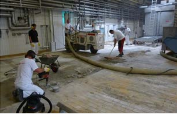
FRIDAY AFTERNOON: Mechanical removal of old tiles and epoxy adhesive. Substrate preparation and cleaning.
