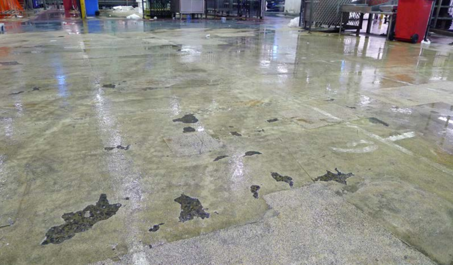
Sydney Fish market before renovation.
