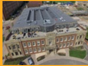
SINGLE PLY ROOFING
