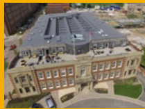
SINGLE PLY ROOFING
