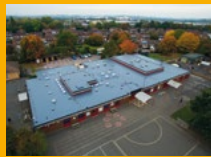
LIQUID APPLIED ROOFING
