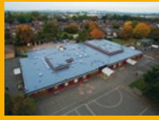
LIQUID APPLIED ROOFING
