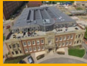
SINGLE PLY ROOFING
