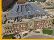
SINGLE PLY ROOFING
