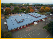
LIQUID APPLIED ROOFING
