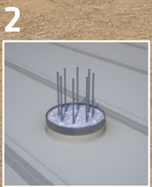
SikaProof® detailing solutions, e.g. for pile caps
