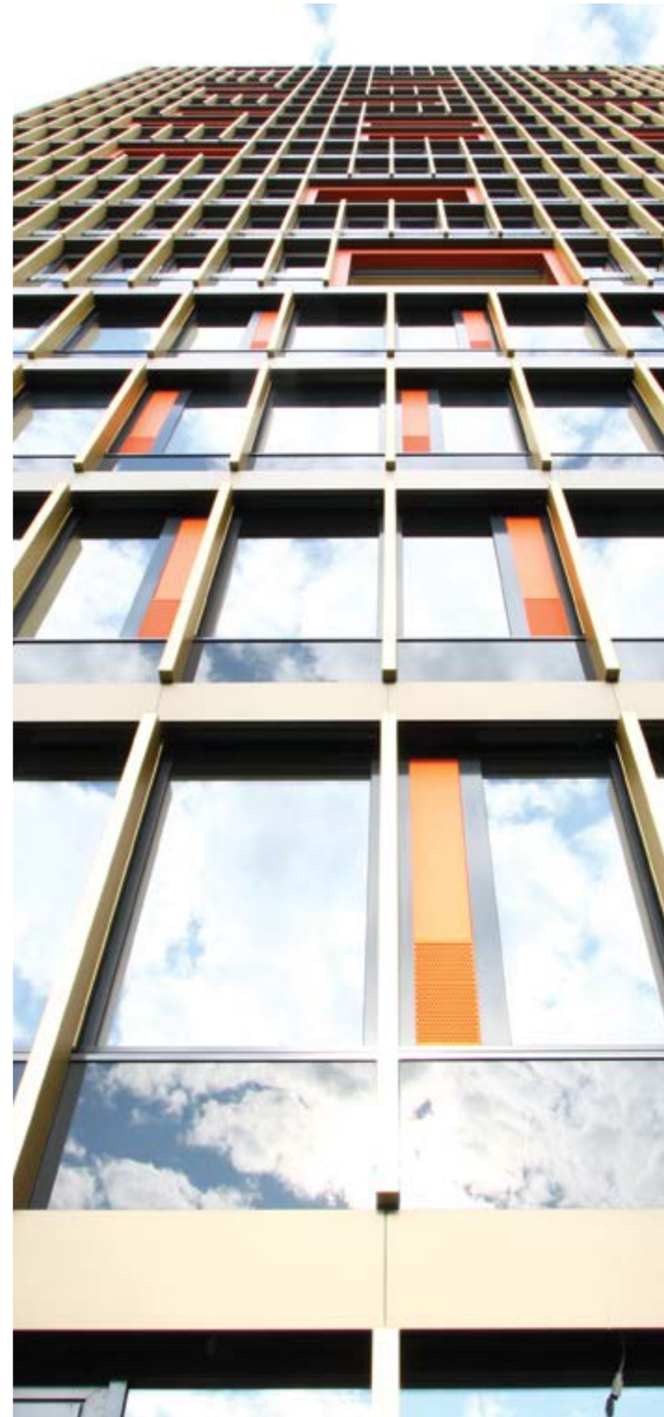
left: Leutschentower, Zurich, Switzerland, 2011 Architect Bétrix Consolascio; Architekten AG, Zurich Window manufacturer Baumgartner AG Window type Wood/aluminum with opening lights bonded with SikaFast®-5201 NT
