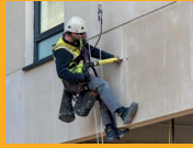
JOINT SEALING
