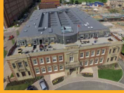
SINGLE PLY ROOFING
