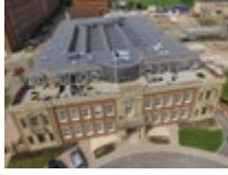
SINGLE PLY ROOFING
