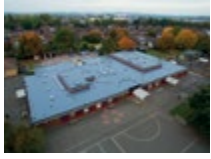
LIQUID APPLIED ROOFING
