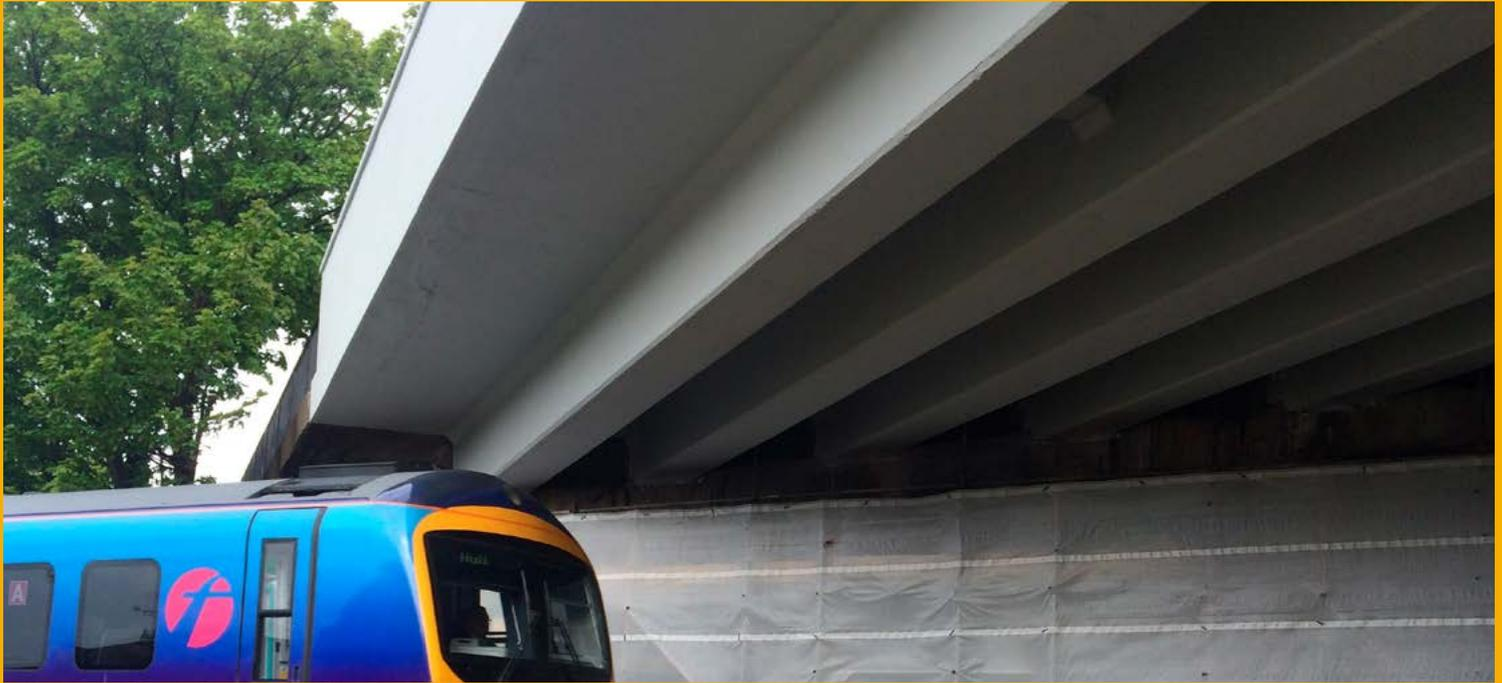
The concrete bridge, built in 1964, displayed major signs of carbonation-induced spalling to columns and deck soffits above the rail lines. Contractors, BOSA Contracts, on behalf of Hull City Council, required a practical repair solution which extended the lifespan of one of the city's arterial routes without impacting on daily road and rail commuter journeys or impeding pedestrians.
