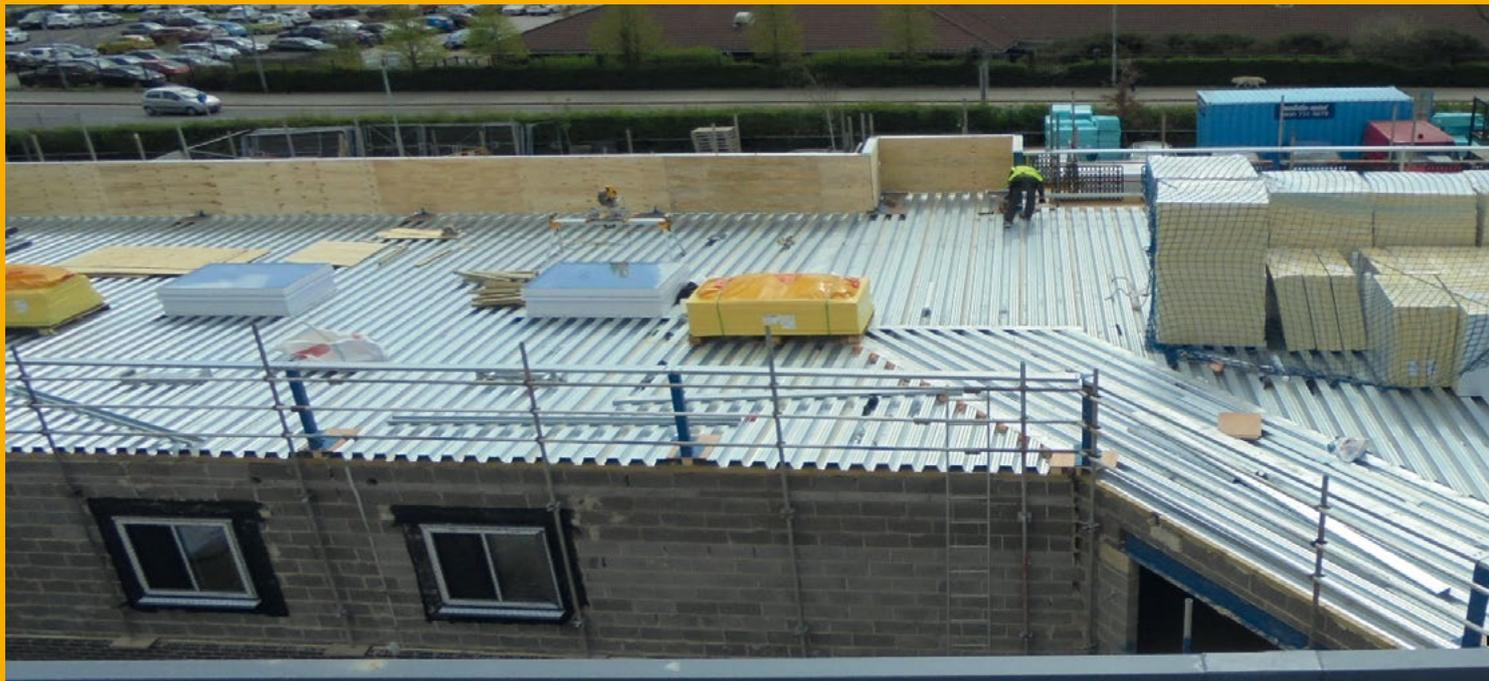
The first phase, which began in January 2017, involved a complex operation to provide a smart, watertight system to an unusually-shaped, multi-directional roof featuring a myriad of details including plant materials and rooflights. For this challenging application, Sika-Trocal® Type 'S' system was selected.
