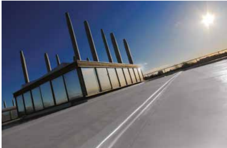
ABOVE: ABERDEEN UNIVERSITY THE ROOF OF ABERDEEN UNIVERSITY'S CHEMISTRY BUILDING WAS THERMALLY UPGRADED USING SARNAFIL AND SARNA THERM INSULATION, REDUCING CARBON EMISSIONS AND ENERGY COSTS.
