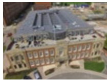
SINGLE PLY ROOFING
