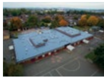
LIQUID APPLIED ROOFING
