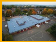
LIQUID APPLIED ROOFING
