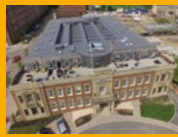
SINGLE PLY ROOFING
