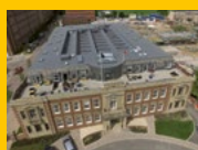
SINGLE PLY ROOFING
