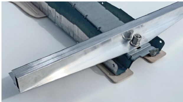
Mount positioning along the chalk lines.
