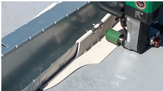
Hot-air welding of a SikaRoof® Click flange with a semi-automated welding machine.
