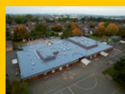
LIQUID APPLIED ROOFING
