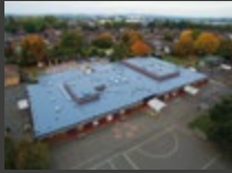
LIQUID APPLIED ROOFING
