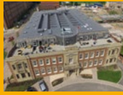
SINGLE PLY ROOFING
