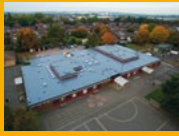
LIQUID APPLIED ROOFING
