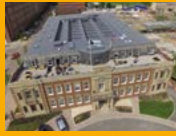
SINGLE PLY ROOFING
