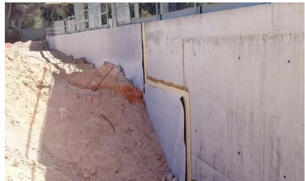
For open excavations: The protection of the SikaProof® membrane is mandatory, especially regarding the backfilling.
