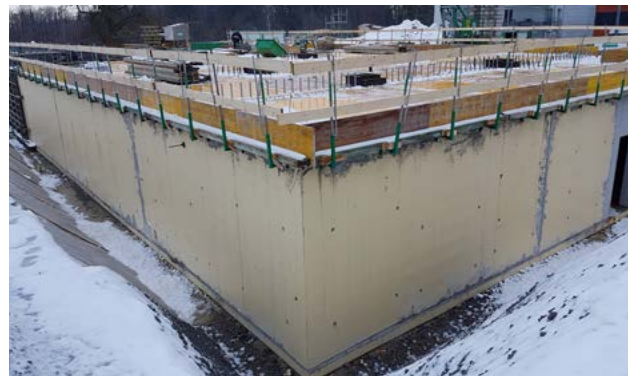
Open excavation with SikaProof® A+: After removing the formwork, the anchor penetrations have to be sealed.
