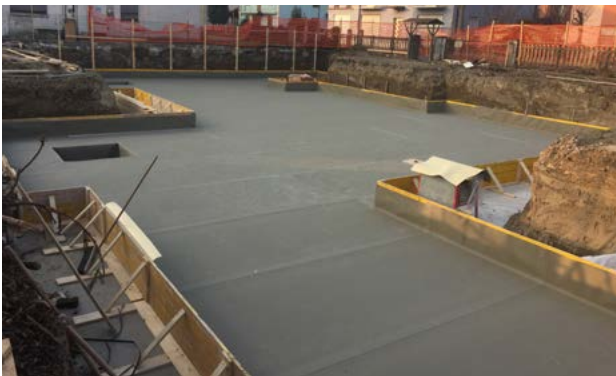
Typical application of SikaProof® A+ on base slab.
