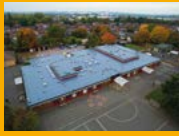
LIQUID APPLIED ROOFING
