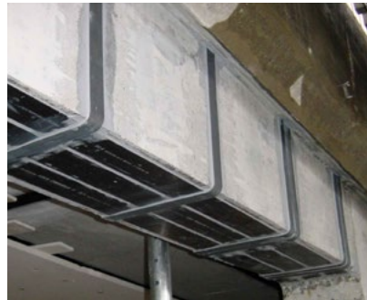
BEAM STRENGTHENING
