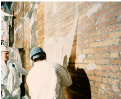
SEISMIC UPGRADING /EARTHQUAKE DAMAGE REPAIR
