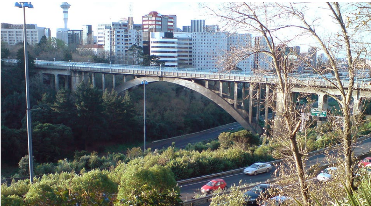
Grafton Bridge, Auckland, New Zealand
