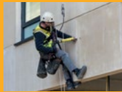
JOINT SEALING
