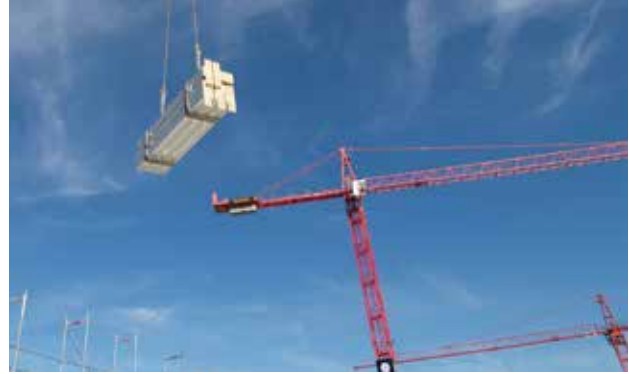
Fast application rate can assist construction programs
