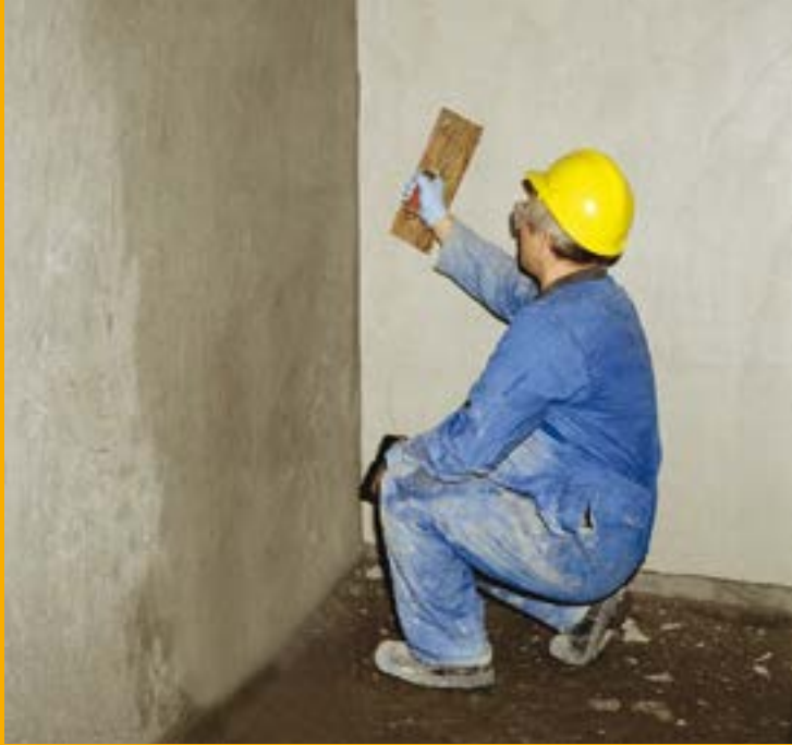
Example of Sika®-1 being applied
