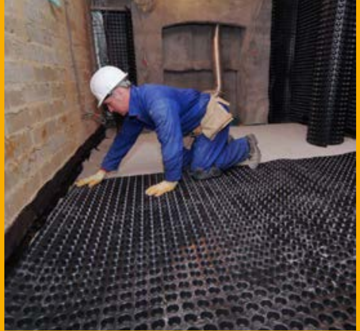
Example of Sika® Cavity Drainage being installed
