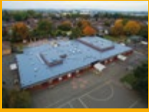
LIQUID APPLIED ROOFING
