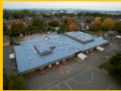
LIQUID APPLIED ROOFING
