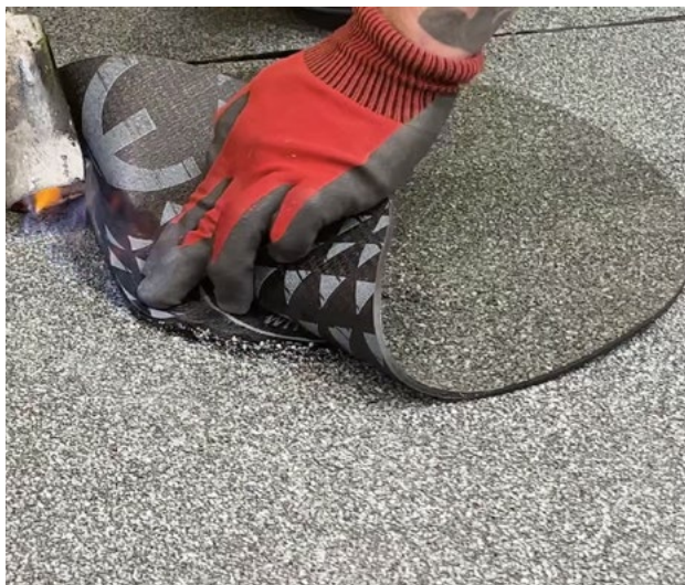
Torch application of the base sheet.
