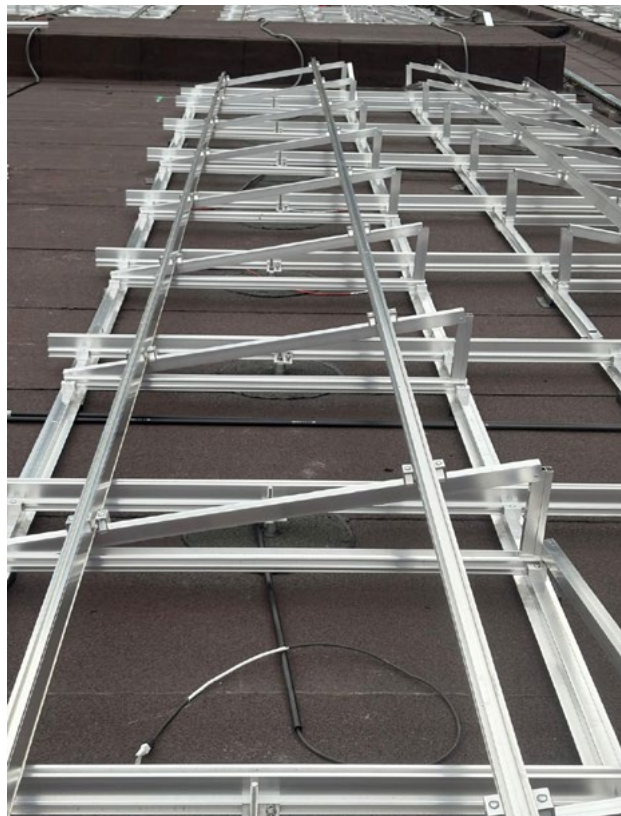
Solar Mounting Systems finalised.
