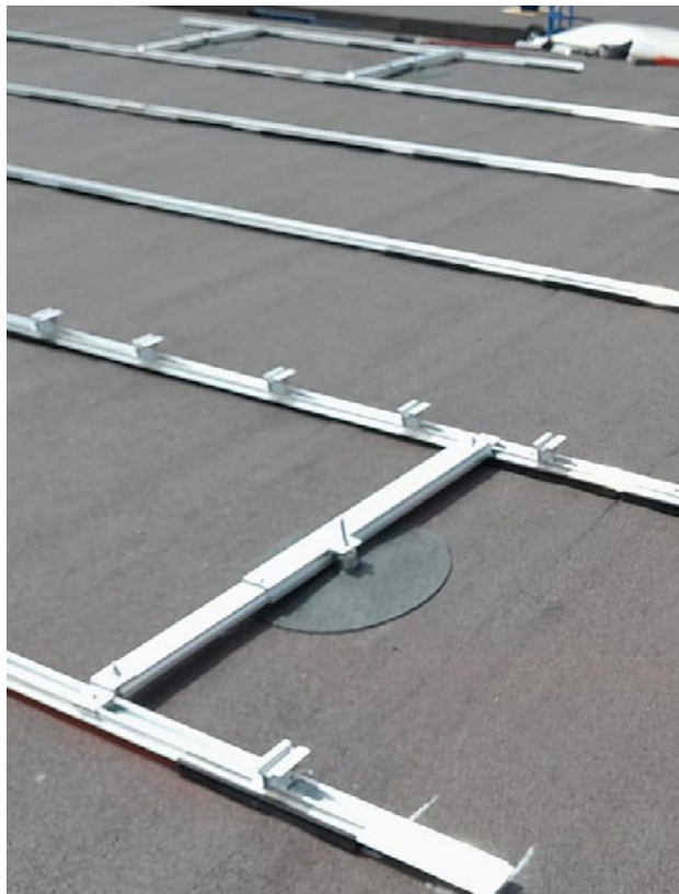
Installation of SikaShield® Anchors and Solar Mounting System.
