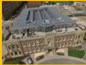
SINGLE PLY ROOFING
