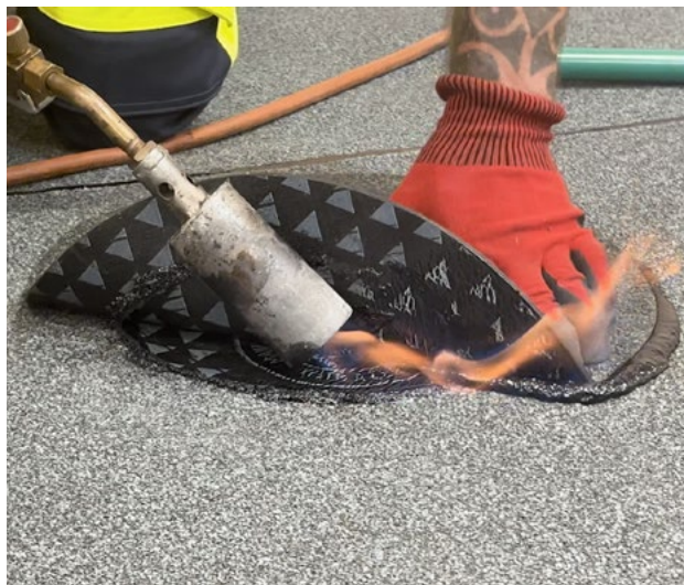
Torch application of the cap sheet.
