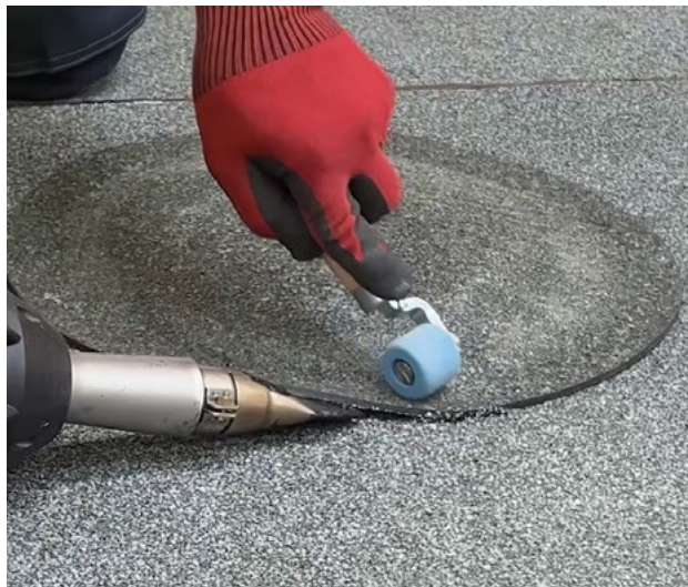
Hot-air application of the cap sheet.
