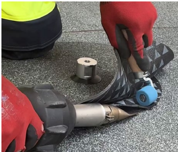
Hot-air application of the base sheet.
