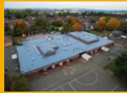
LIQUID APPLIED ROOFING
