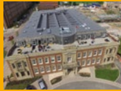
SINGLE PLY ROOFING
