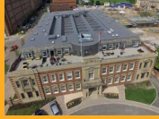
SINGLE PLY ROOFING
