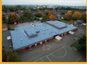
LIQUID APPLIED ROOFING
