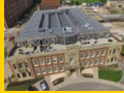
SINGLE PLY ROOFING
