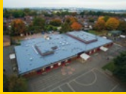
LIQUID APPLIED ROOFING
