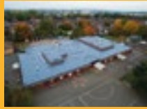
LIQUID APPLIED ROOFING
