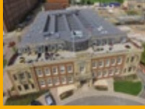
SINGLE PLY ROOFING
