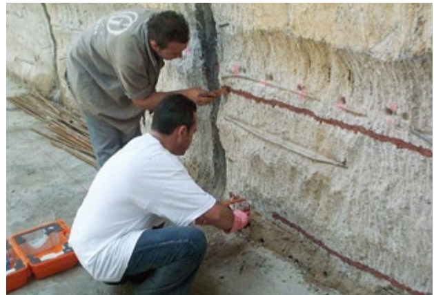
Connection diaphragm walls
