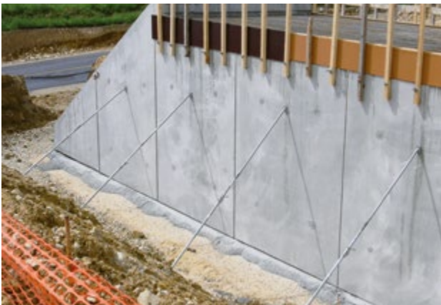
Precast concrete elements
