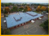
LIQUID APPLIED ROOFING
