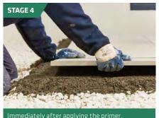
Immediately after applying the primer, lay the paving flag onto the mortar bed
