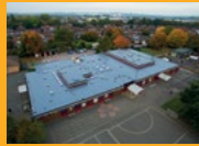
LIQUID APPLIED ROOFING
