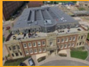
SINGLE PLY ROOFING
