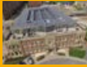
SINGLE PLY ROOFING
