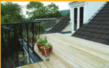
ROOF TERRACES AND BALCONIES
