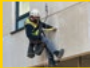
JOINT SEALING
