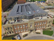
SINGLE PLY ROOFING
