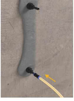
Injecting the crack:
