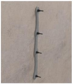
Allow Sikadur Injection Resin to cure minimum 12 hours @ 20°C (68°F)
