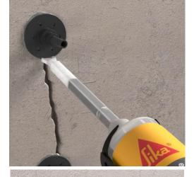
Seal the crack between the ports......
