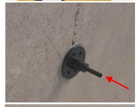
Fix injection ports to crack....
