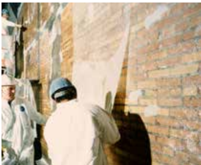
SEISMIC UPGRADING /EARTHQUAKE DAMAGE REPAIR
