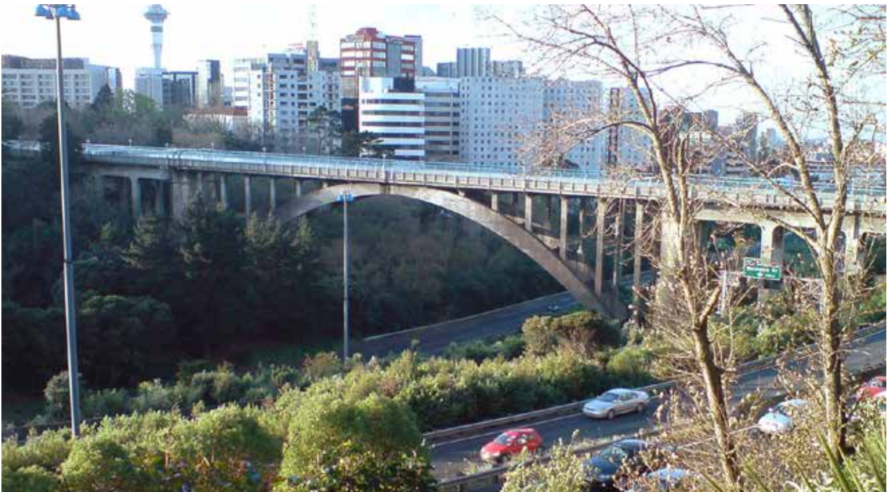
Grafton Bridge, Auckland, New Zealand
