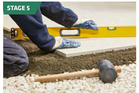
Tap down using a rubber mallet and check flag is level. Cure for up to 72 hours.
