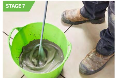
Using an electric mixer, mix until a smooth liquid forms. CAUTION: Adding too much water will cause the mixture to split and make it unusable.
