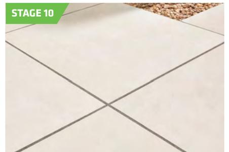
Ensure the product has sufficiently hardened before cleaning the surface of the flags with a sponge and bucket.
