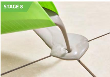
Once mixed correctly, pour the compound into the joints. Pour within 15 minutes of mixing.
