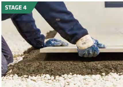
Immediately after applying the primer, lay the paving flag onto the mortar bed.
