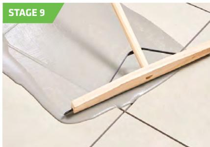
Use a squeegee to guide the jointing compound into exposed joints to obtain fill level.
