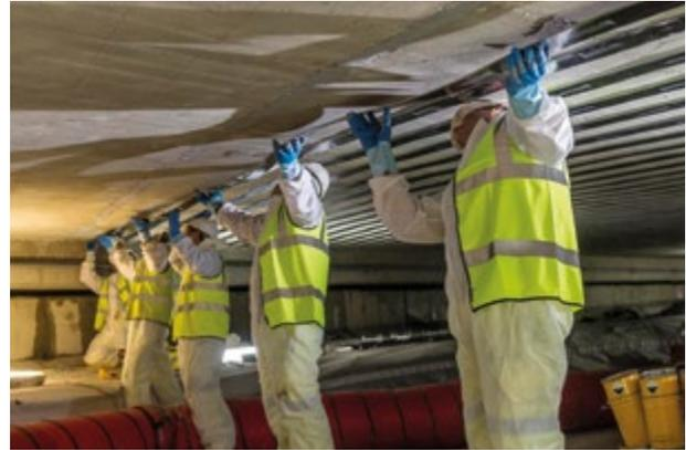
When the M3 Hawley Lane Bridge started to show signs of excessive deflection under heavy traffic, engineers at Enterprise Mouchel devised a repair solution that included the installation of a new central bridge pier to support two existing outer piers. To counteract changes to the deck's dynamics and reinforce the bridge between the three structural piers, Sika® Carbodur® rods and Sika® Carbodur® plates were used – marking one of Europe's largest applications of composite reinforcement systems.
