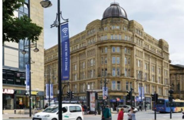
In the heart of Bradford city centre, Britannia House was in need of renovation as its concrete exterior and steel frame was showing signs of failure. With substantial fractures to the stone cladding and corrosion to the steel frame and rebar, Sika provided a complete refurbishment solution including cathodic protection – with more than 2,500 anodes installed across the top three floors.
