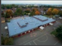
LIQUID APPLIED ROOFING
