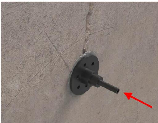
Fix injection ports to crack....
