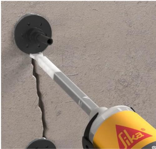
Seal the crack between the ports.....
